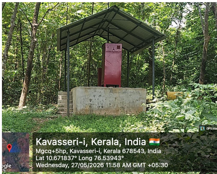
Figure 6: Photograph showing the magazines
